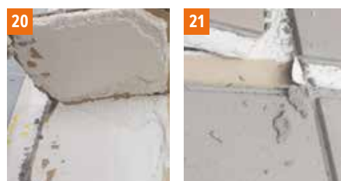
Photos 20, 21 Geoflex Express. Pull-off test of a tile glued on a mortar layer with a thickness of 3 mm after 3 hours - the substrate is destroyed.
